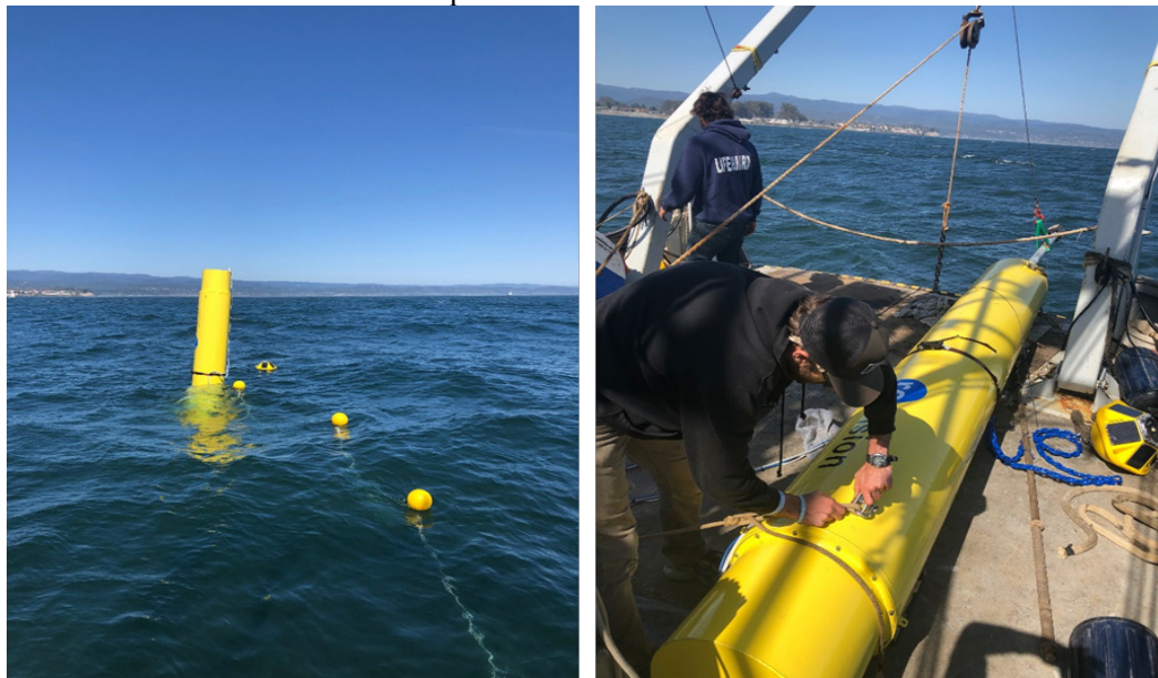
Figure 15 - Buoy deployed at sea (left) and on deck before installation (right)
